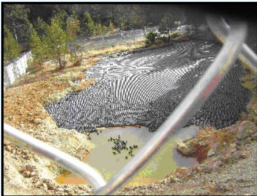
Photo 3: Bird Ball™ installation to protect waterfowl
